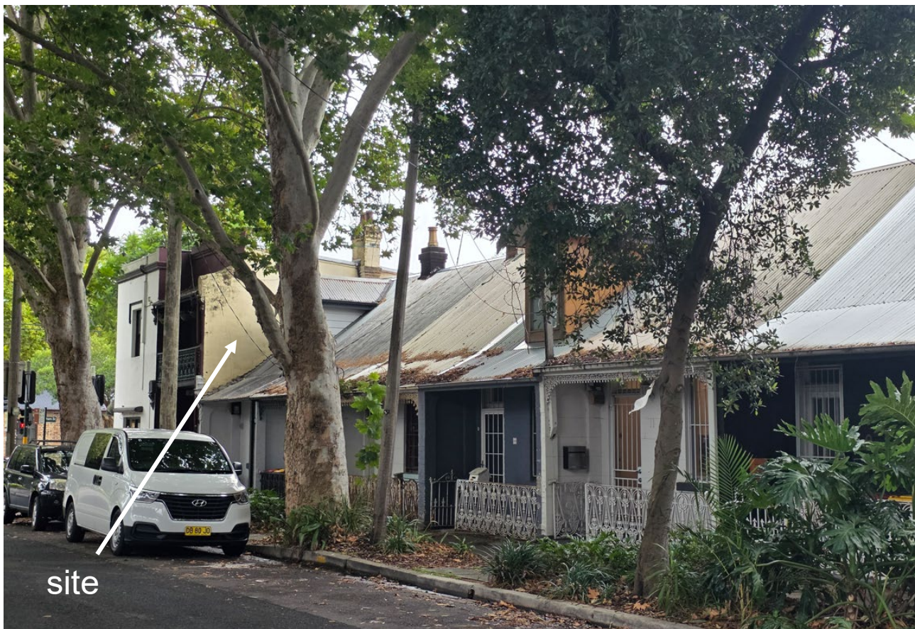
View toward site from Buckland Street facing northwest
