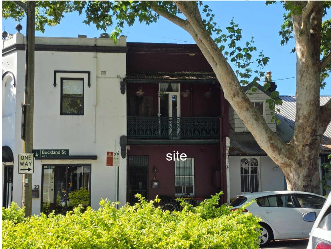
Site viewed from Buckland Street facing north
